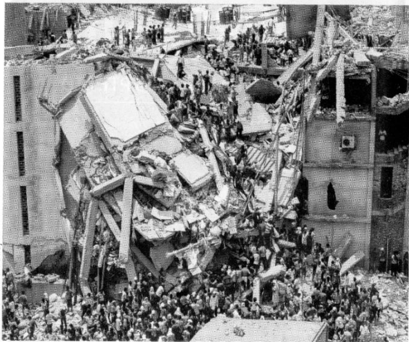
People rescue garment workers trapped under rubble at the Rana Plaza building on the outskirts of Dhaka after it collapsed in 2013.
